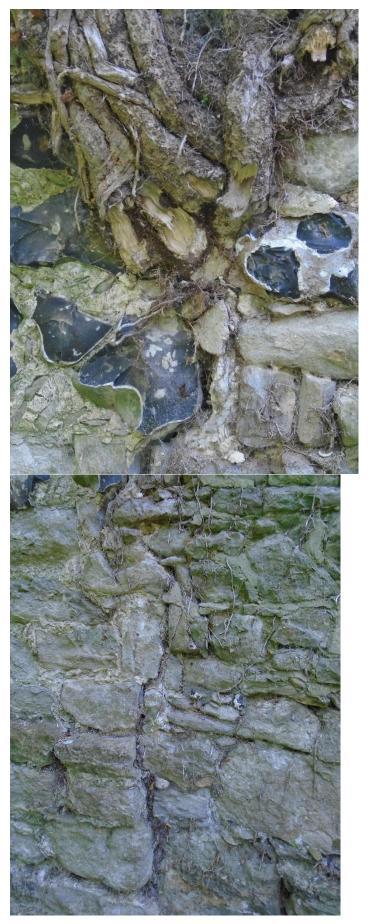
There is a crack that runs from below the cut ivy to ground level but there does not appear to be any safety issues regarding this crack.
