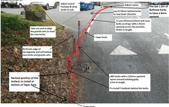
For info, as it stands with the layout of the road, when the gully blocks or during heavy rainfall surface water over runs the ends of the speed ramp, flows into Church Lane and causes flooding issues to property.
